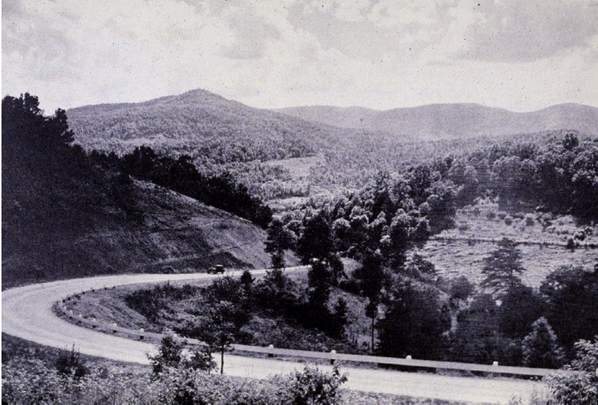
TVA Freeway Near Norris Dam
