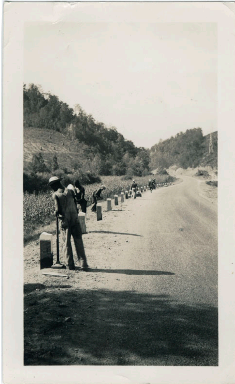
Otto F. Haslbauer, Photographer; Tamping and finishing posts for guard rail along freeway, 1935 (Volunteer Voices: The Growth of Democracy in Tennessee (single images))
