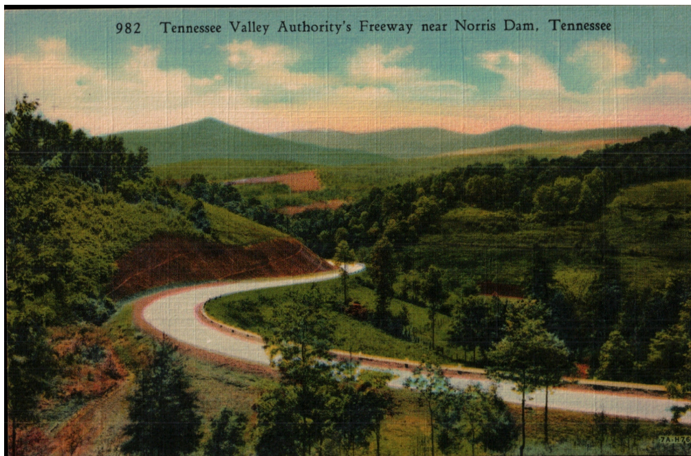
TVA Freeway Near Norris Dam
