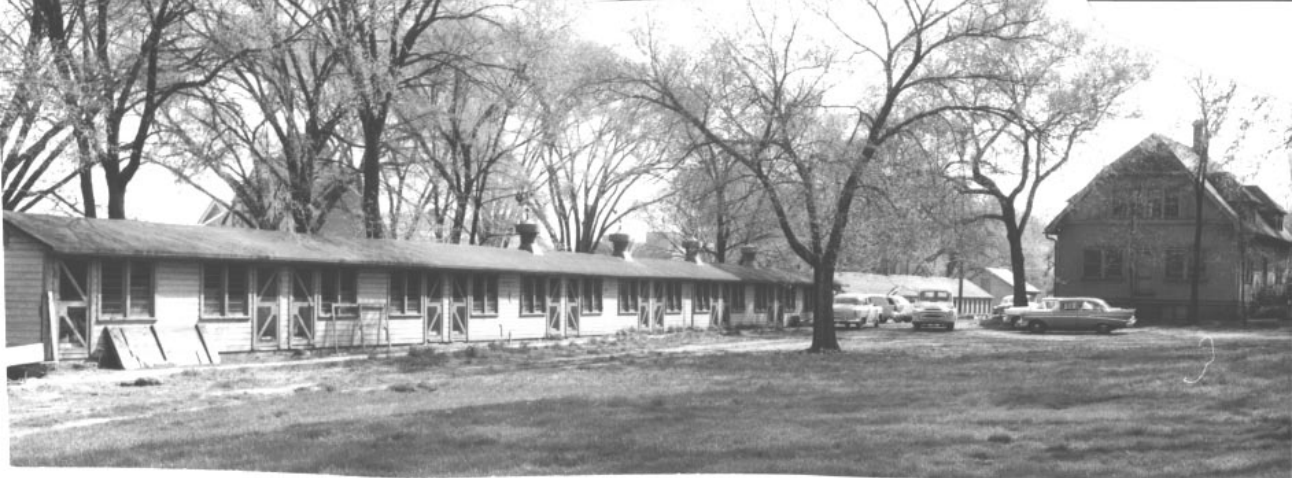
Fig. 1. The poultry building (on the far right) with associated "long houses" before its reincarnation as a rehabilitation facility and sea grant administration offices. 1969. [series 9/3 Poultry Houses, jf-36]
