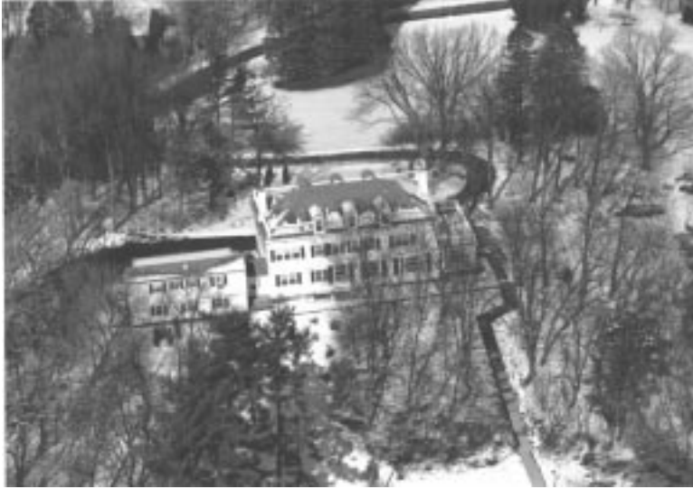
Fig. 1. 1997. The President's house, with new garage at left.. The remodeling included not only bringing the house up to modern building codes, but the construction of a garage with living quarters, and sun room. [Del Brown photo, AP-79]
