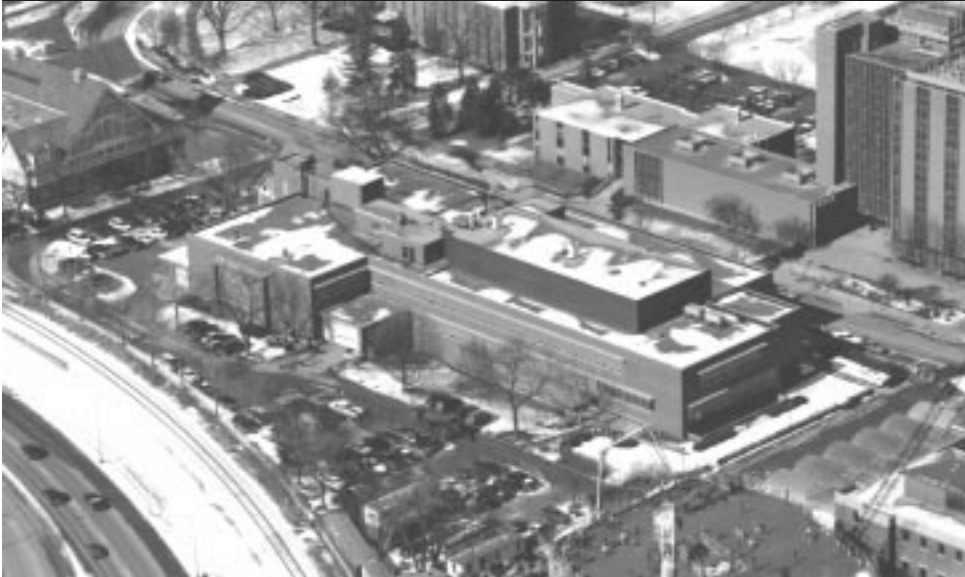
Fig. 1. Babcock Hall after the 1990 addition. [Del Brown photo, AP-81]
