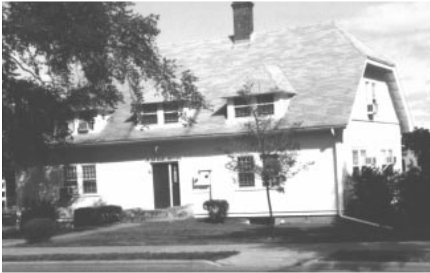
Fig. 2. The Seagrant building from the south side of University Avenue in 1993. [Author Photo AP-4]
