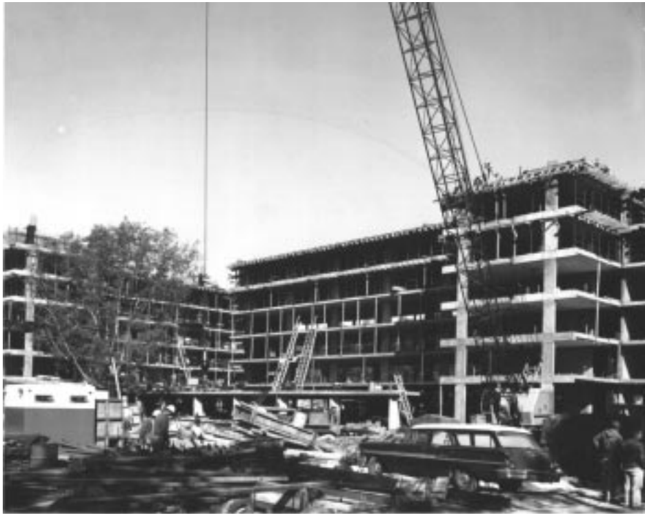
Fig. 2. The first of the southeast dorms going up: Sellery Hall Under construction, September 24, 1962. [Series 26/1, Southeast Dorms, ns-1734]
