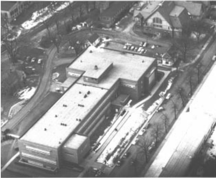
Fig. 3. Air view of Babcock Hall as completed in 1952. [Series 8/5, jf-65]
