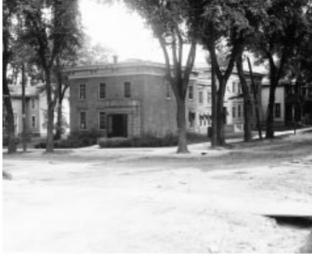
Fig. 1. The Porter House looking SE c. 1890. [series 9/2 administration, old, x25-1338] .
