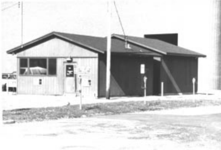
Fig. 1. The Fleet car office and garage, with the Stores building in the background. [Author Photo, AP-57]
