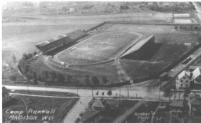
Fig. 3. 1910 The original stadium at Camp Randall. The intersection in the foreground is Randall (left to right) and Johnson Streets. University Avenue is in the extreme upper right. The camera is looking west toward Breese Terrace. The grandstand is at the left. The bleachers on the right were condemned. [series 9/10 Camp Randall, x25-1872]
