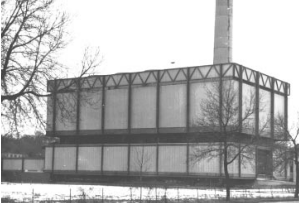
Fig. 1. West Heating plant 1994. [Author Photo, AP-54]
