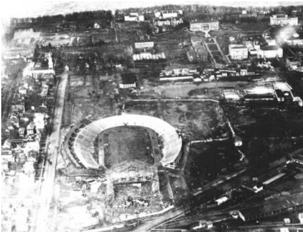
Fig. 2. 1930, the field house is born into the west campus. The steel framework rises to the south of the stadium. Breese Terrace (with trolley cars) is at the left. The recently completed Van Hise dorms and Lake Mendota are in the far background. Note that the engineering campus is almost entirely undeveloped, only the old forest products lab, and the "old sawtooth" engineering lab building (which within two years would be the site of mechanical engineering) are shown. [Series 9/11, M111]
