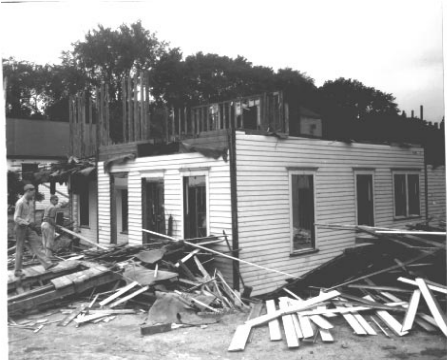
Fig. 3. August 1949, the first dairy building is demolished to make way for Babcock Hall, named for the man who built this building. [9/3 First Dairy School folder jf-13]
