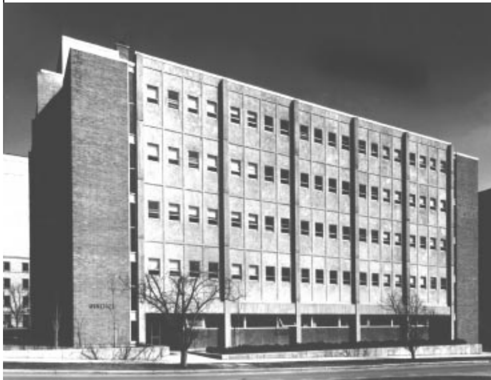
Fig. 1. Genetics building c. 1965. 72 by 128 feet, five stories of precast concrete curtain wall panels, face brick and a gross size of 53,000 square feet. The 1995 biotechnology center connected at the right of this picture. [series 9/3, Genetics, jf-78]
