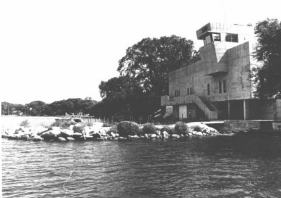
Fig. 1. The Lifesaving Station 1970. The breakwater is at the left; the observation and mechanical decks cantilever towards the lake. [Series 9/2, Lifesaving Station, jf-105]
