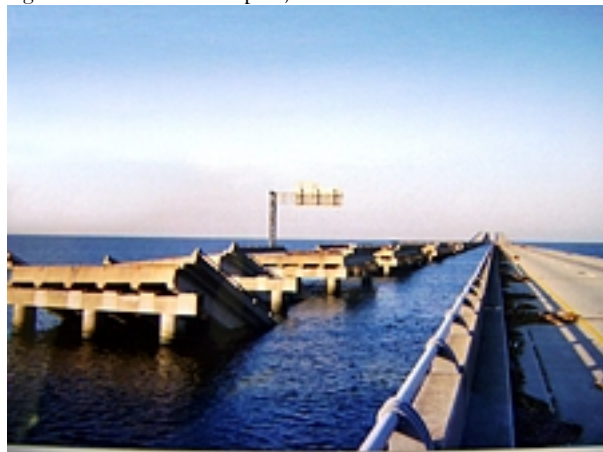
Figure 1.8: I-10 Twin Span, Post Katrina.
