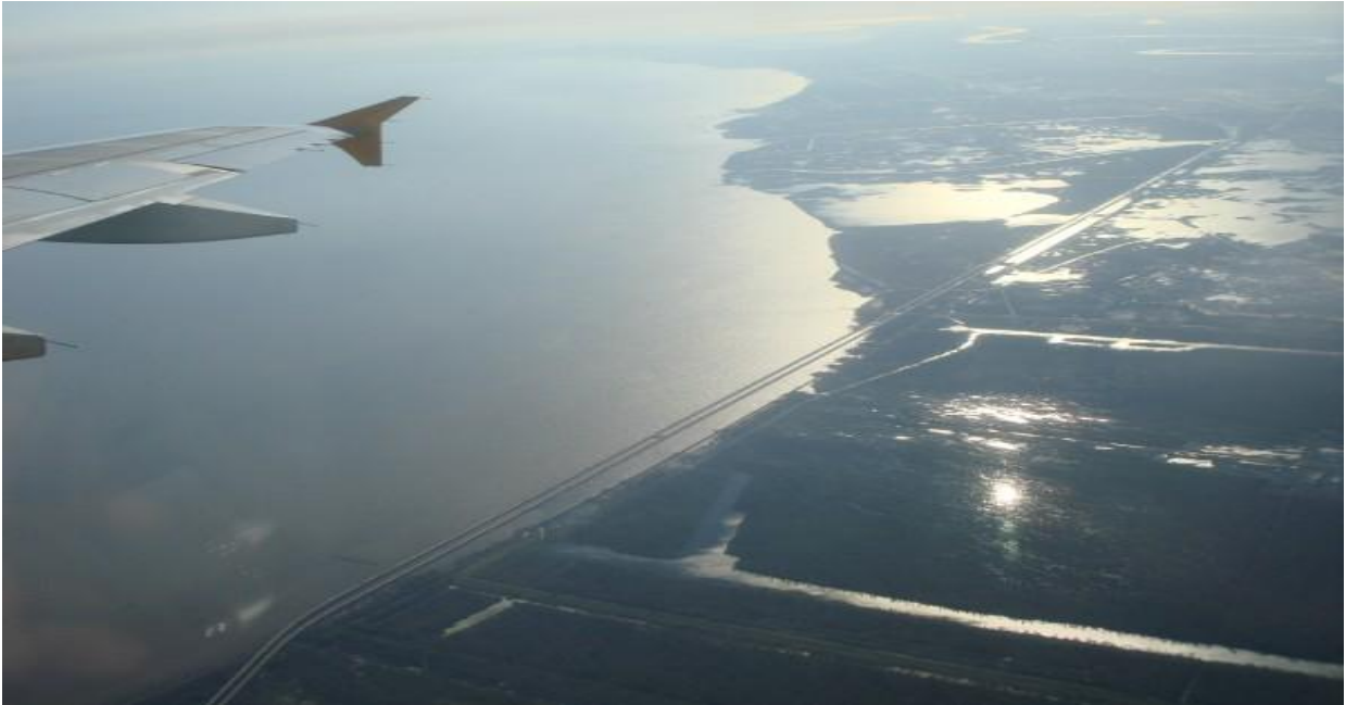
Figure 1.7: Aerial View of The Bonnet Carré Spillway Bridge.
