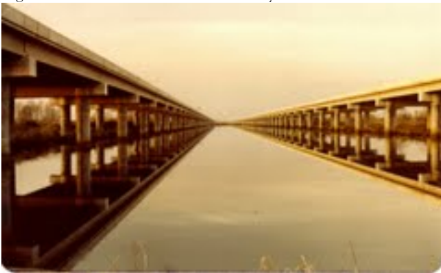
Figure 1.6: I-55 between the causeways.
